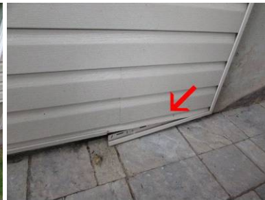
Loose section of siding noted
