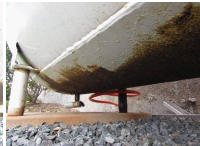
Rust noted on the bottom of the oil tank
