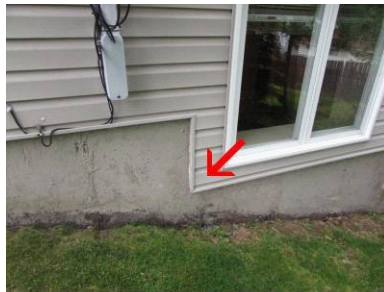
Loose section of siding noted
