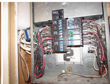
Main electrical panel appears serviceable
