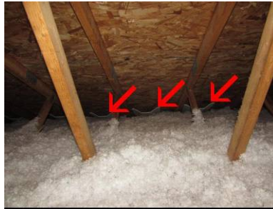
Styrofoam true vent air channels
