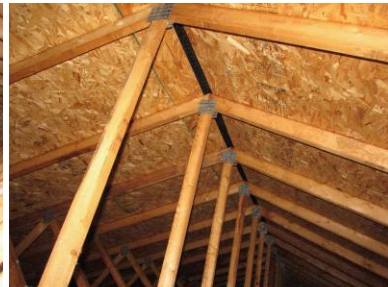
Truss and roof decking system
