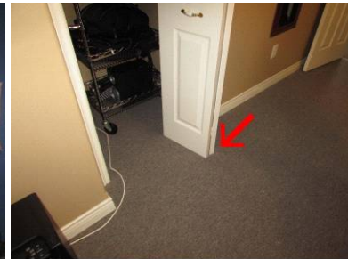
Closet doors bind on the floor
