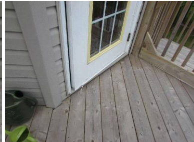
Recommend upgrading door sweep
