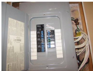
Main electrical panel appears serviceable
