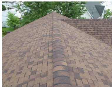
Roof covering appears serviceable
