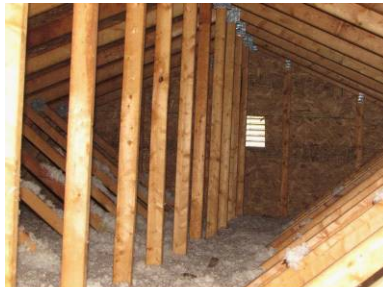
Truss and roof decking system
