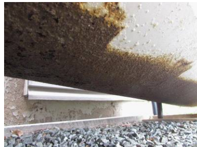
Rust noted on the bottom of the oil tank
