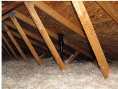
Truss and roof decking system
