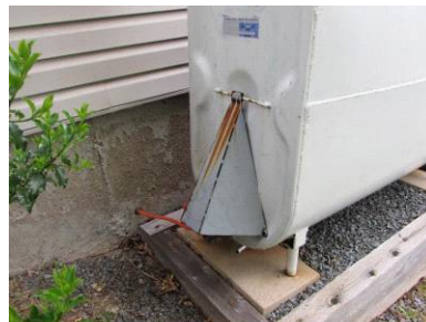
Oil line & valve appear serviceable.
