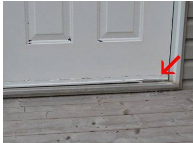
Recommend upgrading door sweep
