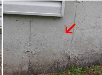
Hairline crack in the side foundation wall
