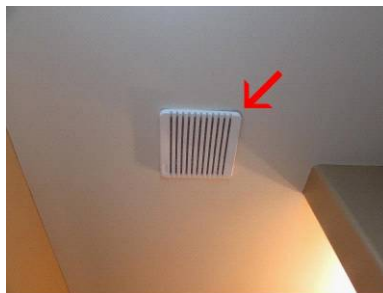
Bathroom ventilation fan requires cleaning
