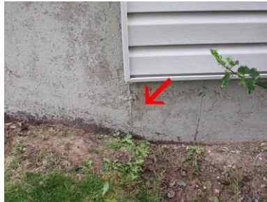
Hairline crack in the side foundation wall
